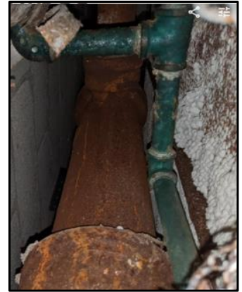
Example of condensation on the cold-water supply pipes.
