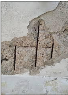
Exposed Rebar
