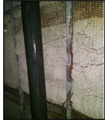
Example of condensation on the cold-water riser.
